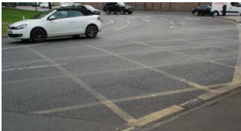
Repainting the yellow boxes at the Grapes Hill roundabout would discourage traffic blocking the exits
