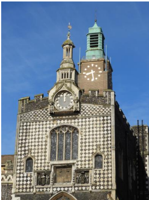
City Hall clock - regularly maintained : Guildhall clock - not working
