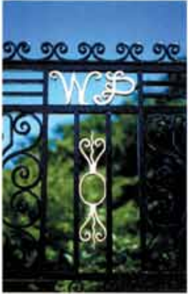
detail of the restored gate on Drayton Road
