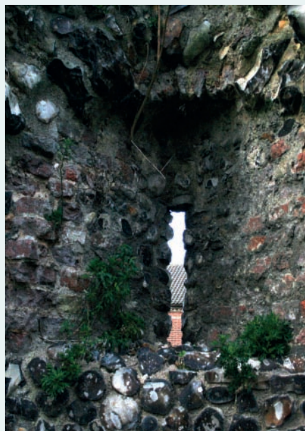
Close-up of an aperture for firing arrows in section of wall at St Martin's at Oak. Photograph:
